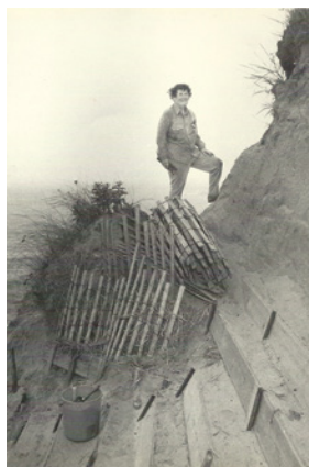
Giordina Reid stands by the shoreline protection system that she designed and helped build to save the Montauk Point Lighthouse.
