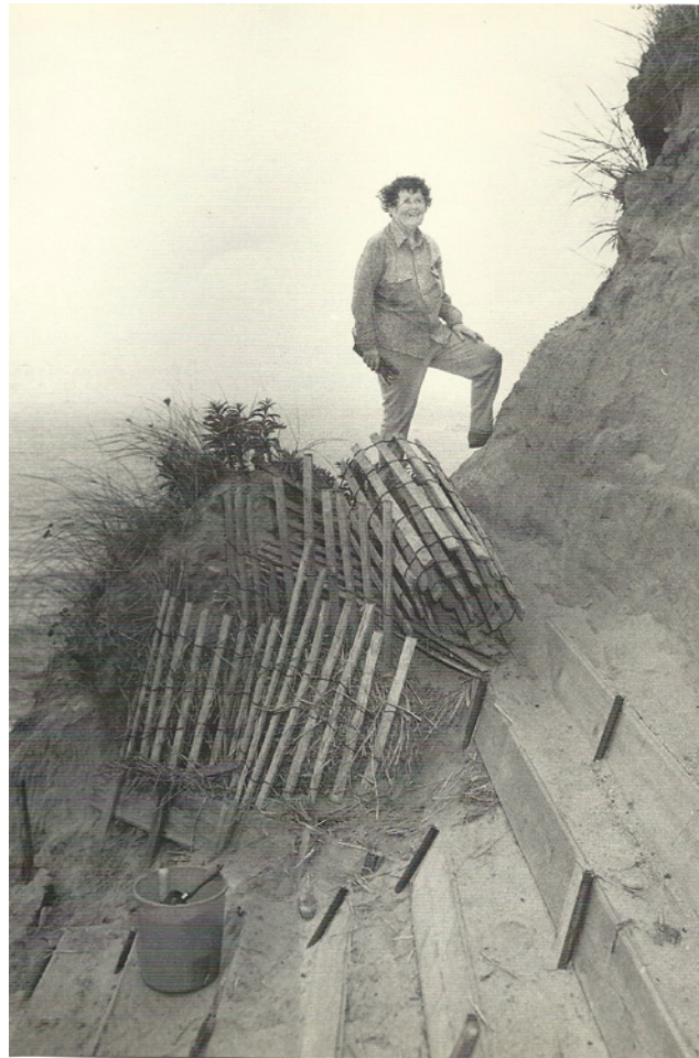
Giorgina Reid stands by the shoreline protection system that she designed and helped build to save the Montauk Point Lighthouse.
